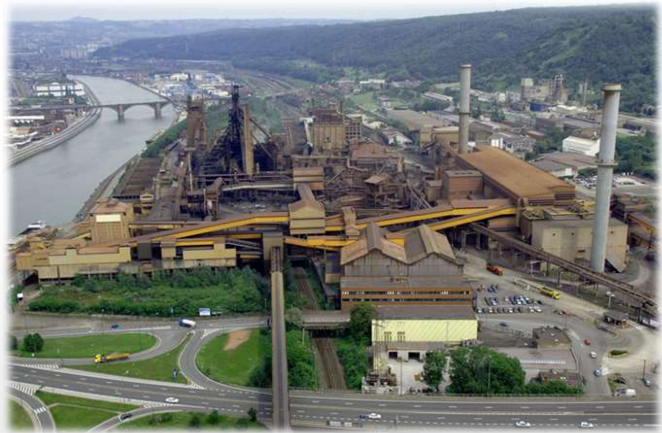
HFB Blast Furnace in Ougrée
